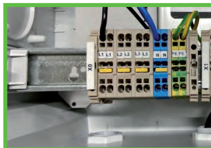
Figure 14 A: 230V connection PURE
